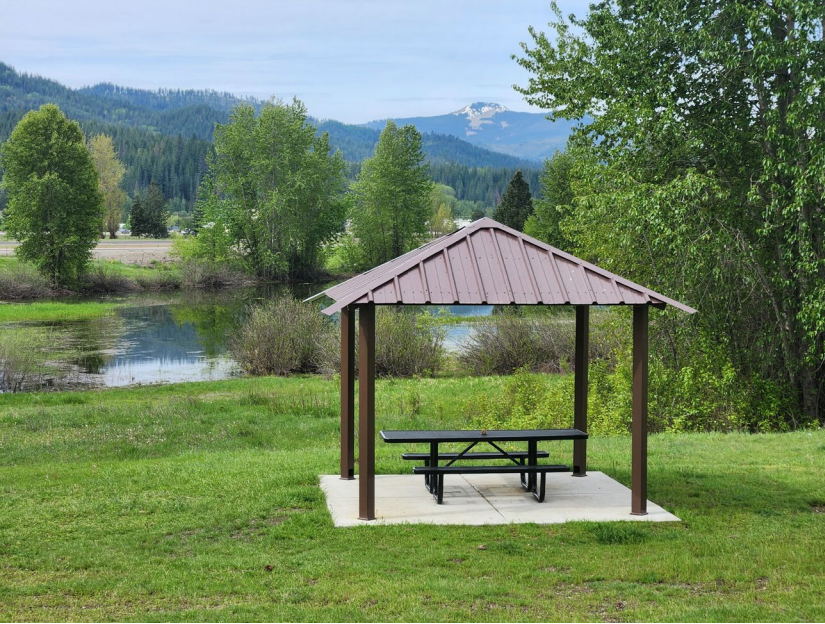
Shade Structure – Kootenai Realtor's Assoc.
