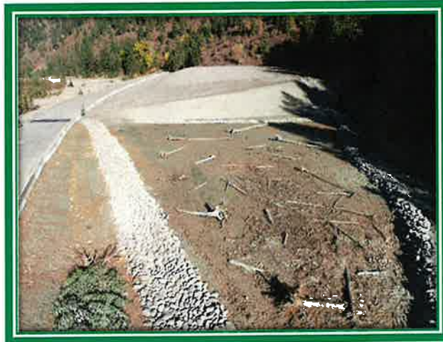
Douglas Complex during following excavation and site grading. Image provided by the CDA Trust.
