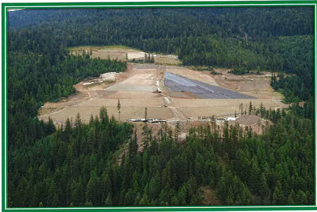
East Fork Ninemile Waste Consolidation Area final cover installation. Image provided by the CDA Trust.
