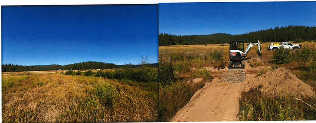
Noxious weed treatments (left), Excavator work for erosion control(right).
