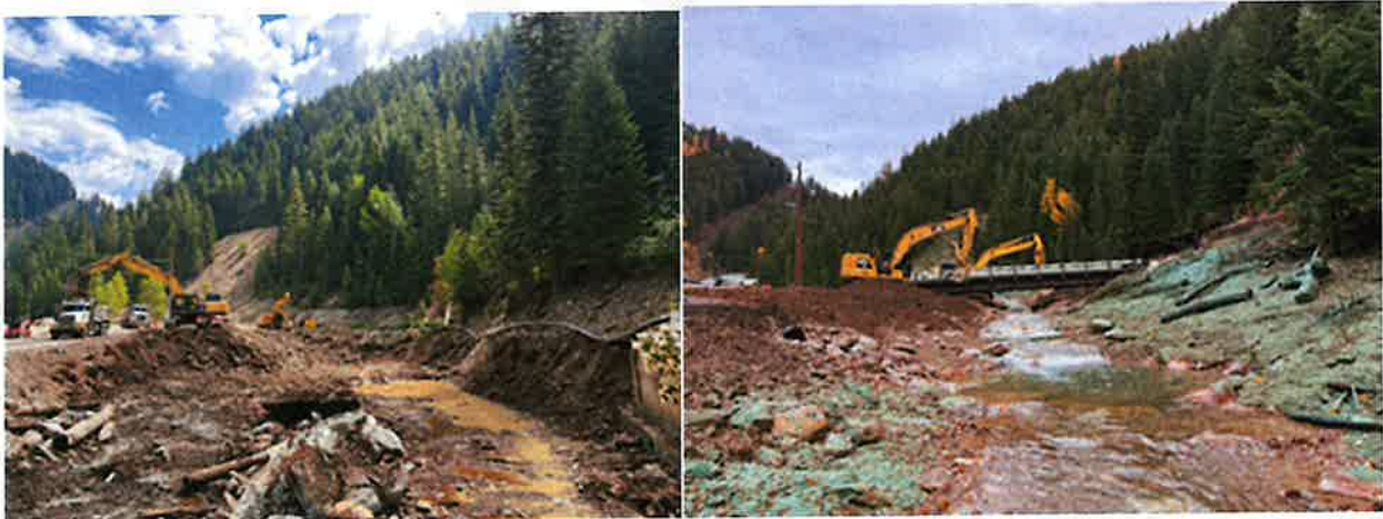
Star Complex during waste excavation (left) and after site grading and stream reconstruction (right). Images provided by the CDA Trust.
