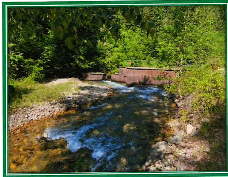
Big Creek fish passage barrier
