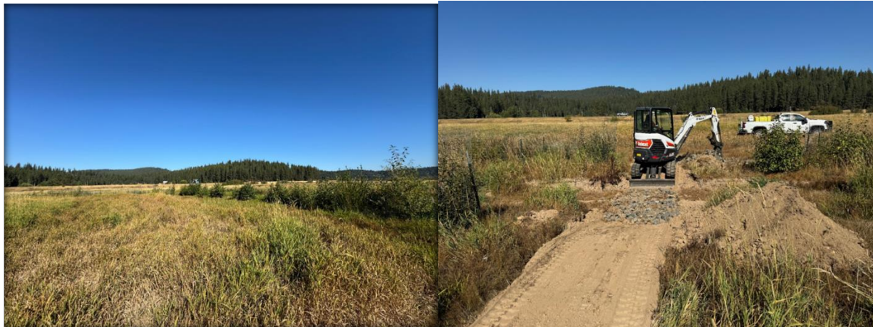
Noxious weed treatments (left), Excavator work for erosion control(right).
