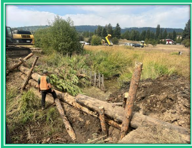
Construction of an instream structure designed to emulate the flow obstruction effects of natural wood jams and beaver dams
