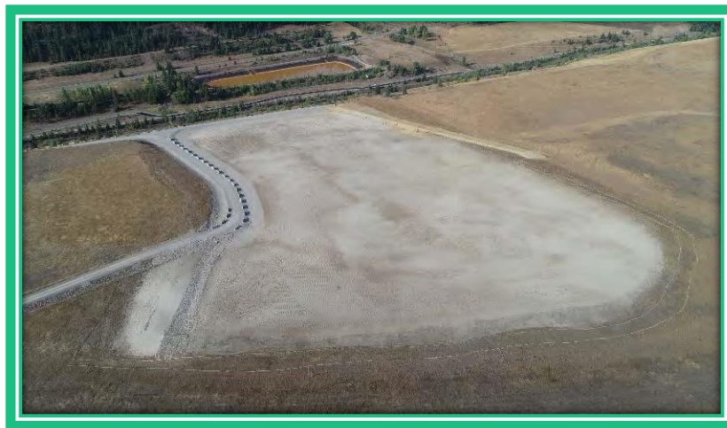
Capped Sludge Pond looking southwest. Photo courtesy of DEQ.
