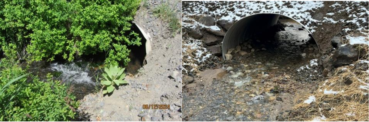
East Fork Bozard Creek culverts before (left panel) and after (right panel) construction
