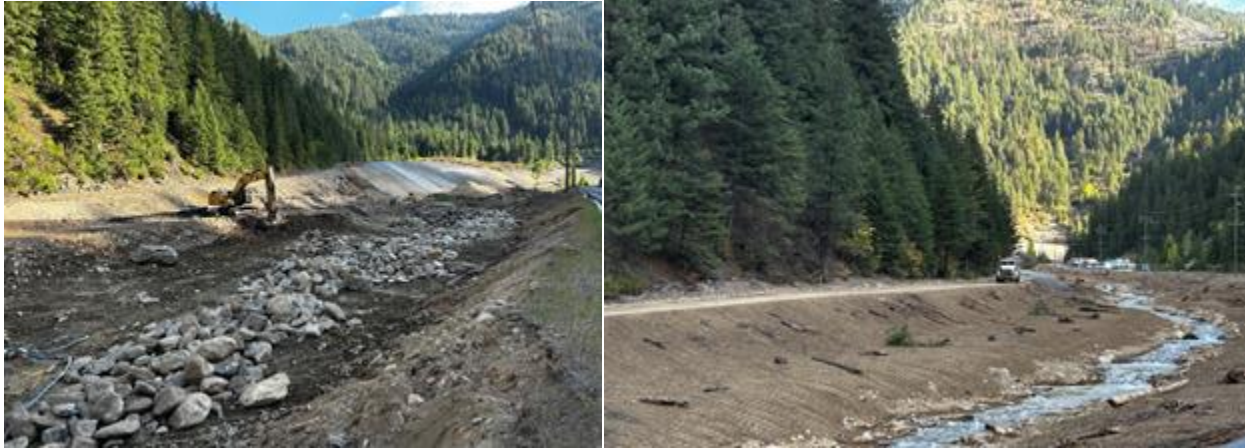
Tamarack No. 7 during waste excavation (left) and after site grading and stream reconstruction (right). Images provided by the CDA Trust.
