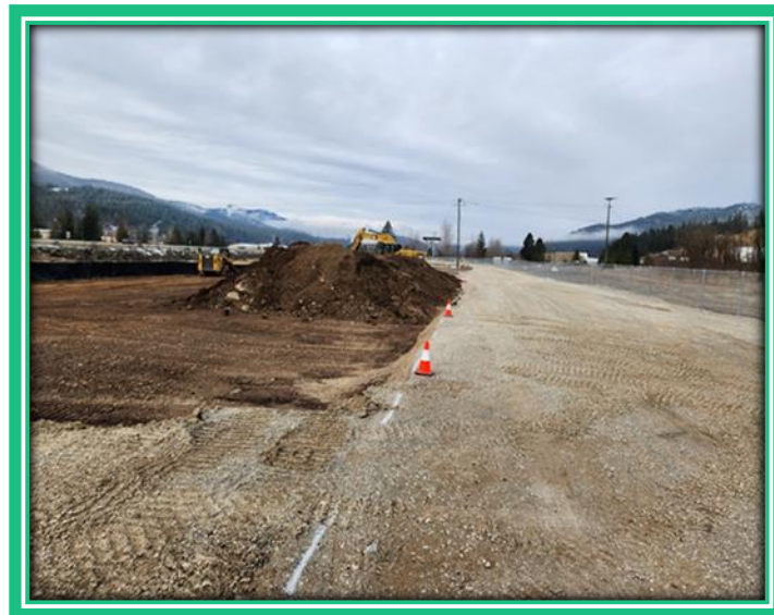
Facing west showing excavation of top foot of contaminated soil along south edge of Theater Bridge Road. Photo courtesy of Idaho Department of Environmental Quality.
