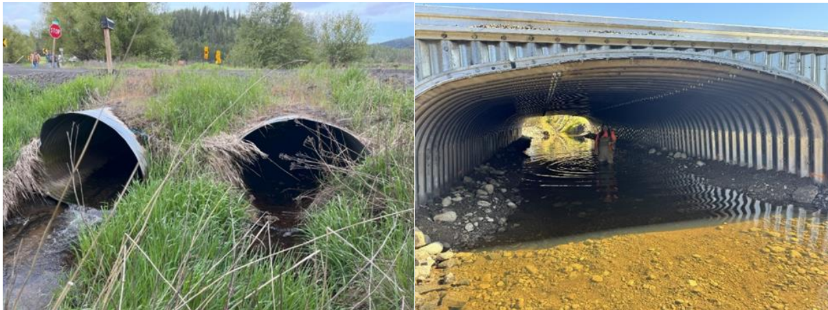
West Fork Lake Creek culverts before (left panel) and after (right panel) construction.
