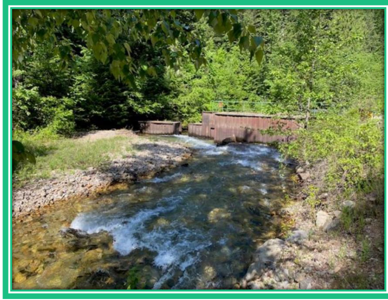
Big Creek fish passage barrier
