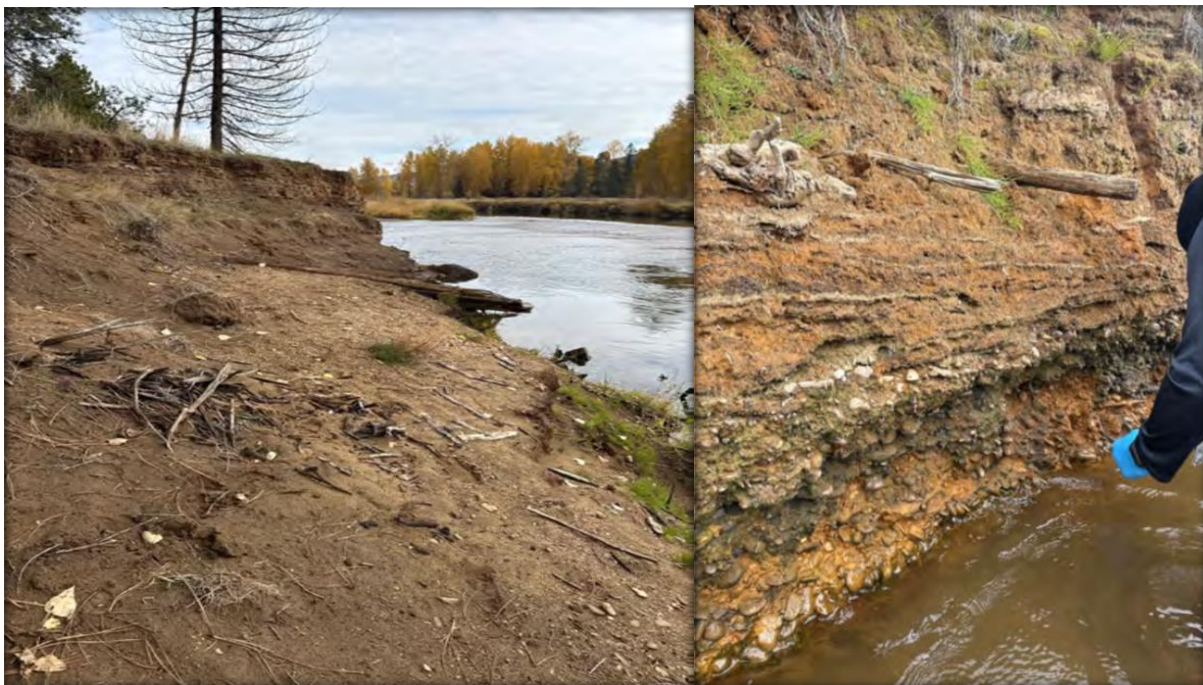
River Mile 165.9 – 167.1 Riverbank Design Focus (Left) River Mile 160 Riverbank Near Cataldo Mission Boat Launch Cataldo Riverbank Pilot Project (Right). Photo courtesy of CDA Trust.
