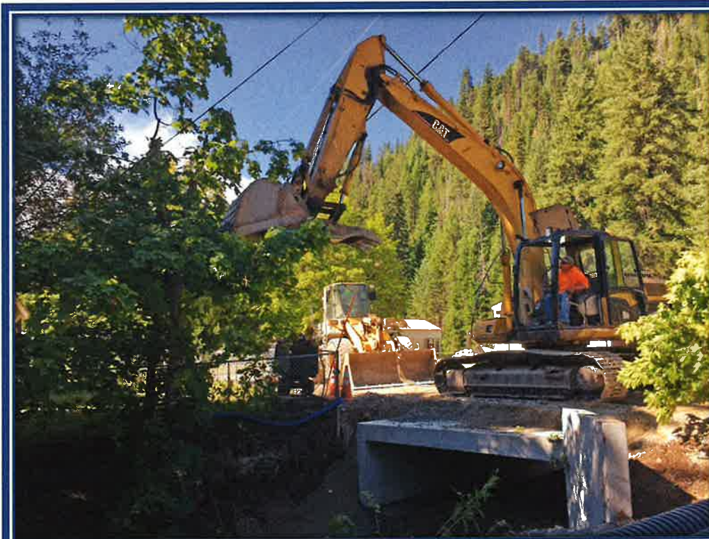
Installation of Fish Passage Bottomless Structure on Black Cloud Creek Project Ninemile Road
