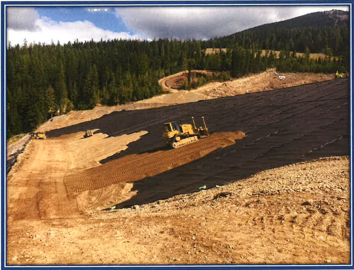
Placing Cover Material Over Final Liner on WCA in EFNM Canyon
