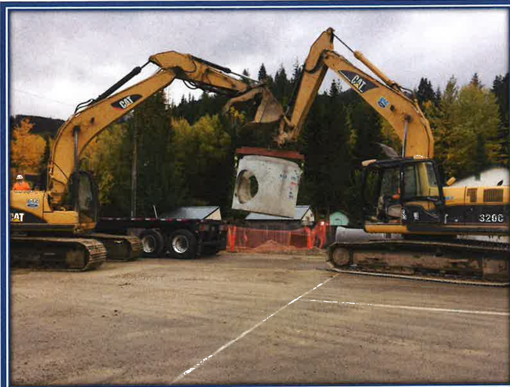
Lifting Large Manhole For Installation on Tiger Creek Project Mullan
