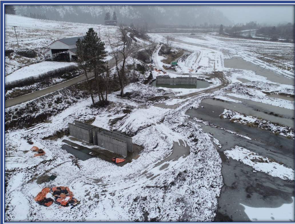
Water Control Structures under construction in the Cave Lake Wetland of the Gray's Meadow Project
