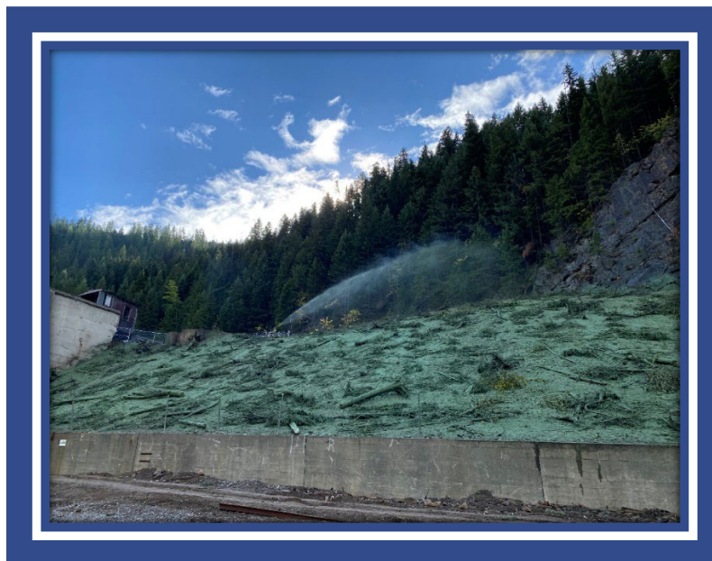
Hecla-Star hydroseed application. Images provided by the CDA Trust.
