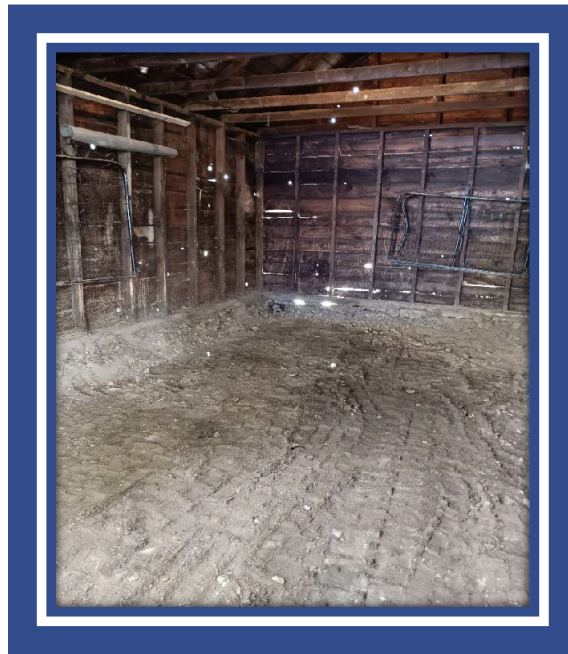
Inside garage. Excavating up to 12-inches. Photo used by permission of the Coeur d'Alene Trust.
