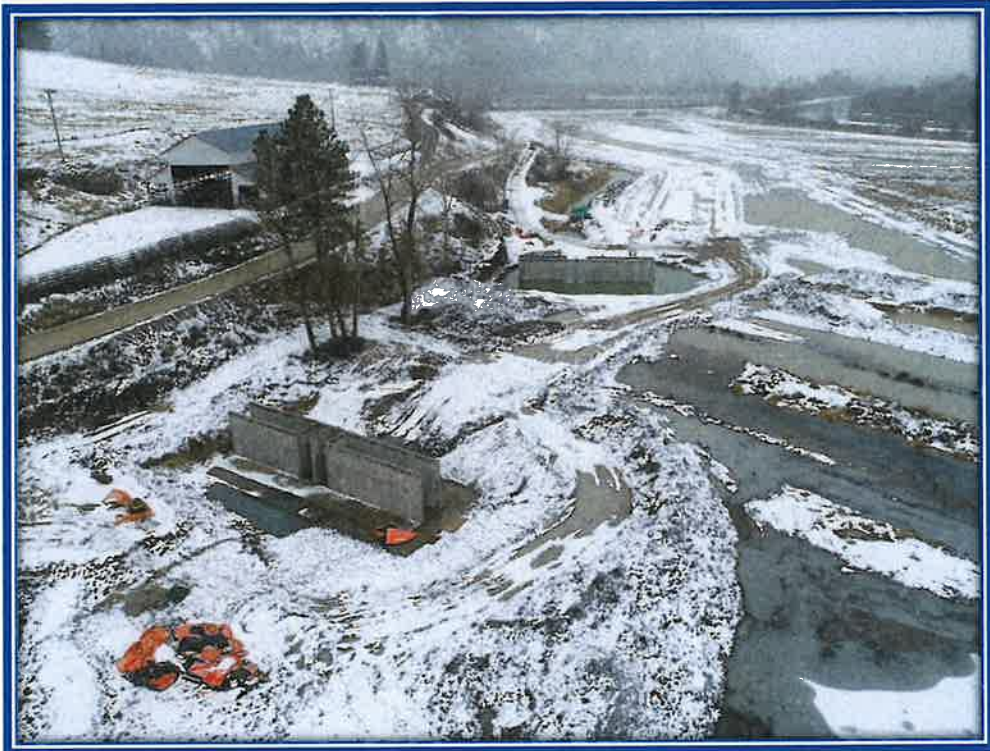
Water Control Structures under construction in the Cave Lake Wetland of the Gray's Meadow Project
