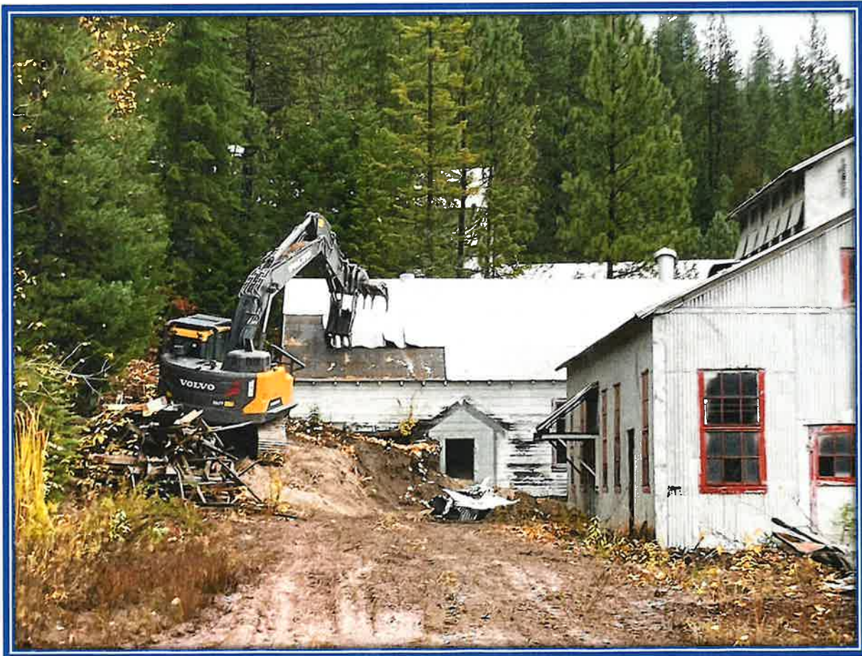
Building Removal Operations Day Rock Complex
