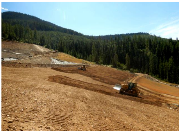
Placing lime-amended soil atop liner system.
