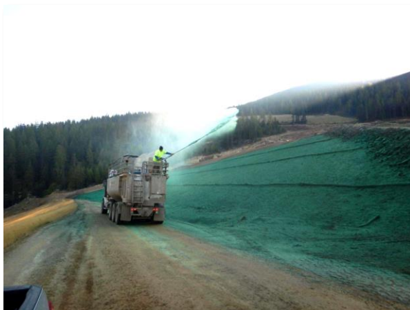
Applying bonded fabric material North Slope
