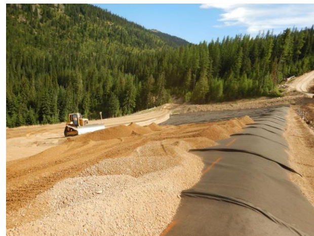
Layering 1"-minus cushion material atop liner system.
