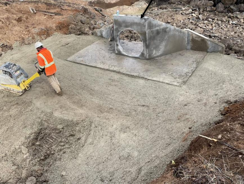
Gravity Discharge Outlet Installation
