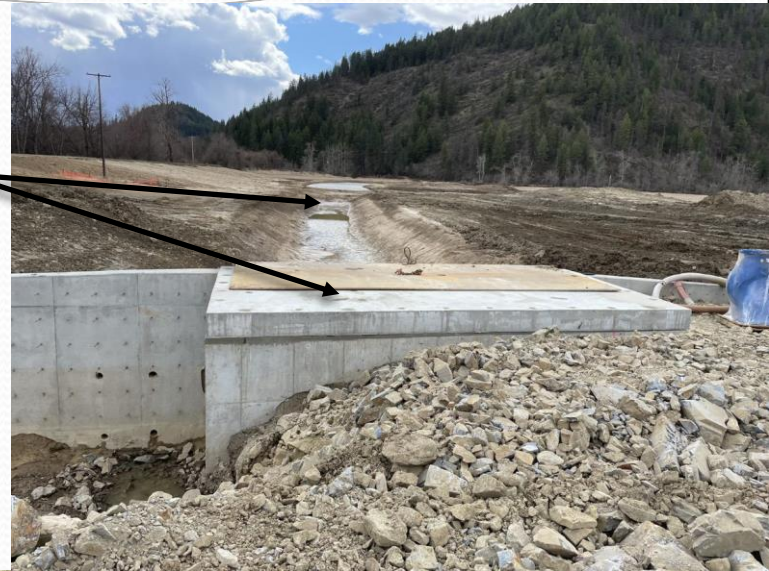
Floor for Pumphouse and Conveyance Channel
