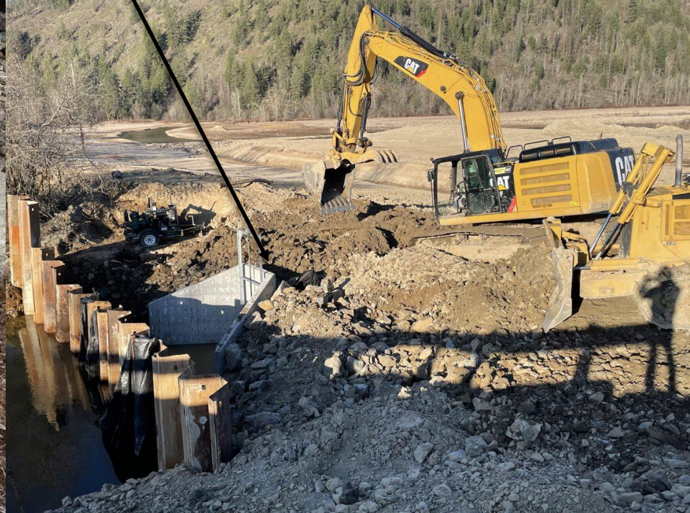
Gravity Discharge Outlet Installation
