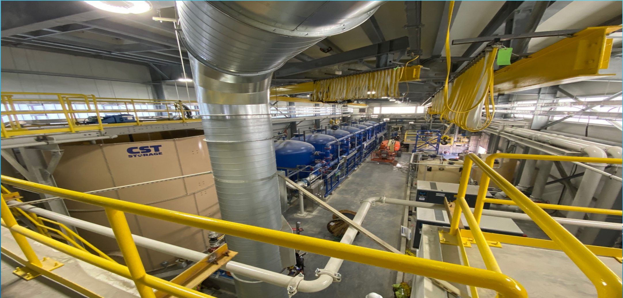
INTERIOR FILTER BLDG. – FILTER VESSELS, DIRTY BACKWASH TANK, POLYMER TANK
