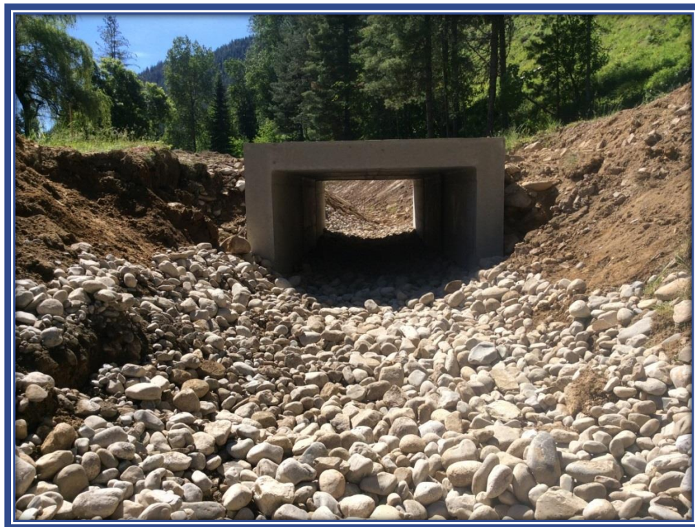
Installation of Fish Passage Structure Rosebud Creek Remedy Protection Project Osburn
