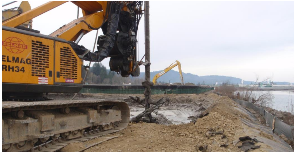
Column mixing using augur for ISS
