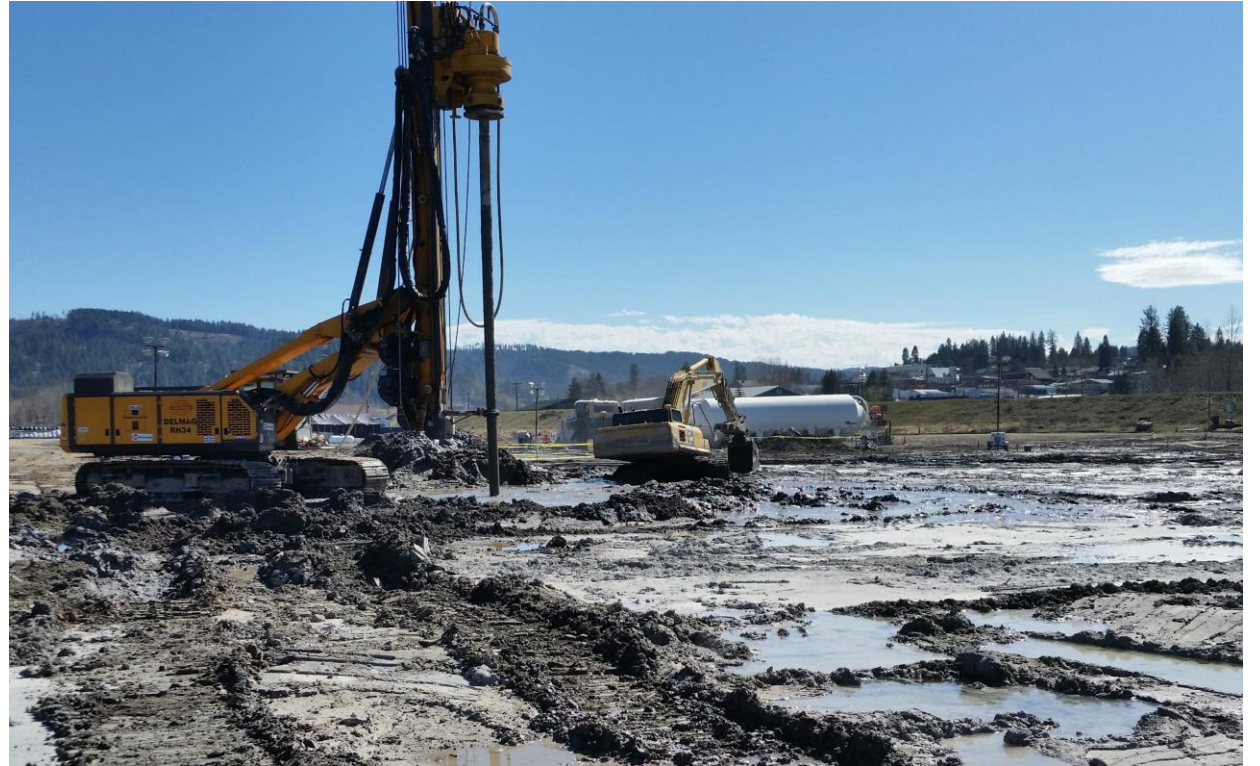
In Situ Stabilization of Impacted Soils to 60'
