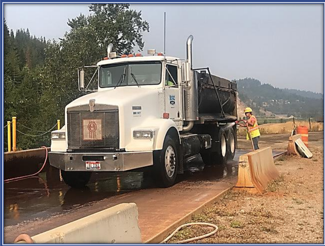
Typical Truck Decontamination After Dumping at Repositories
