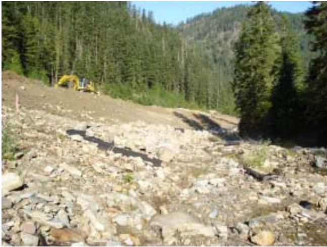
Workers regrade tailings pile to improve stability
