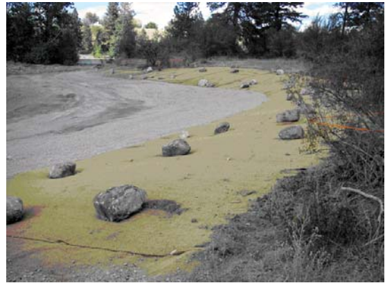
Island Complex: Bank stabilization area
