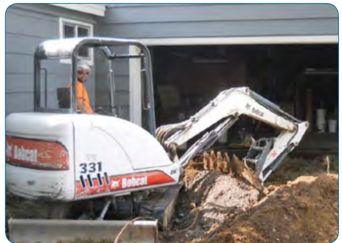
“Refusal flip” remediation in progress this summer.
