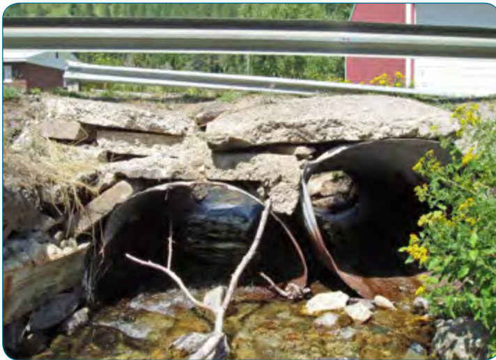
Culverts on Boulder Creek at School Street will be replaced.
