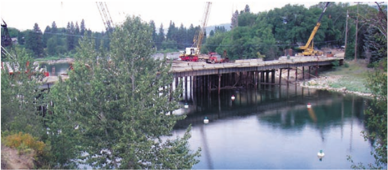
Bridge Under Construction at Barker Road South
