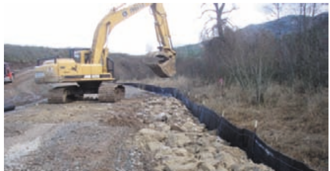
An extra layer of stone was placed along the perimeter of the expansion as rip rap against high flows in Humboldt Creek.
