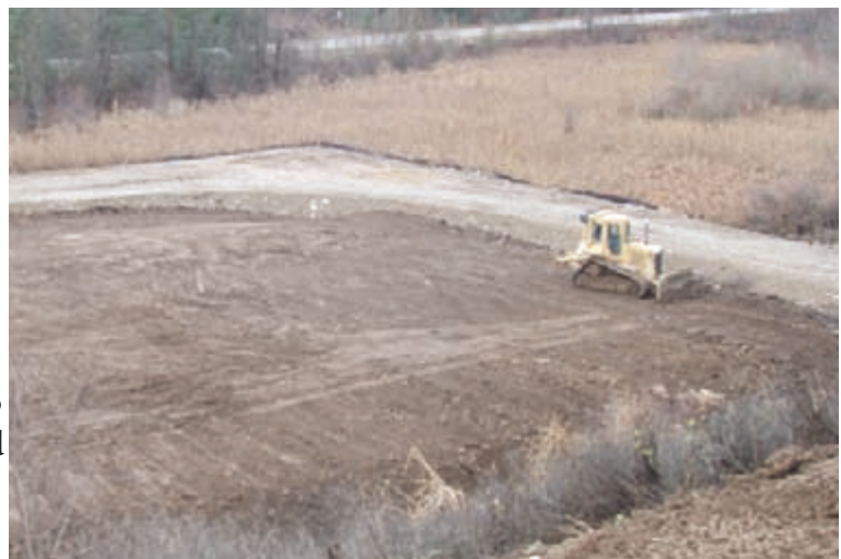
Constructing foundation for Page Repository expansion, fall 2009.
