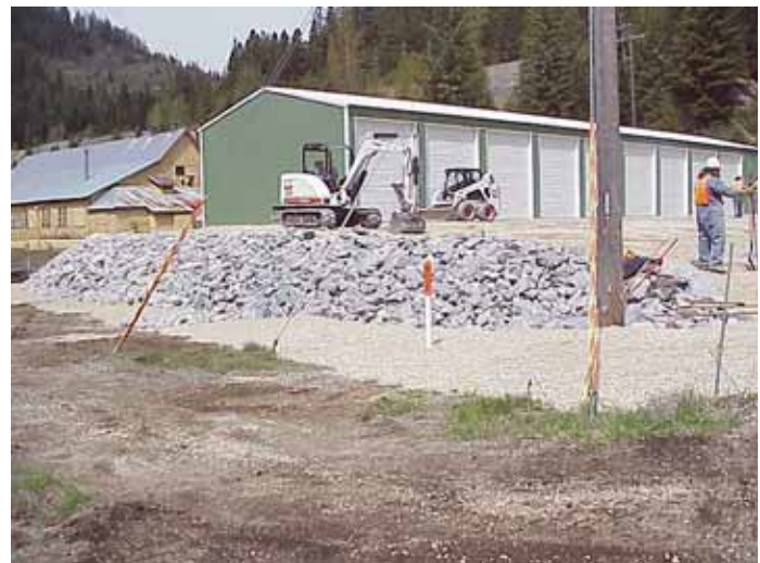
Construction crews removing lead-contaminated soil from properties in the Coeur d'Alene Basin
