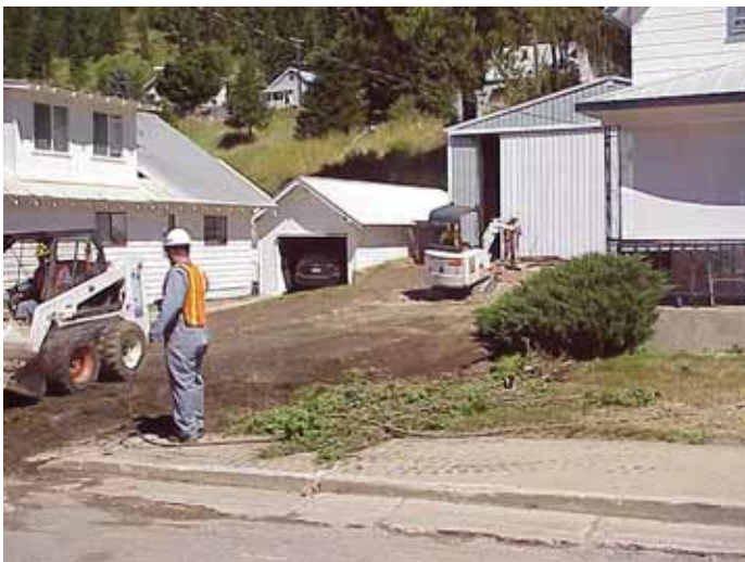
Construction crews removing lead-contaminated soil from properties in the Coeur d'Alene Basin
